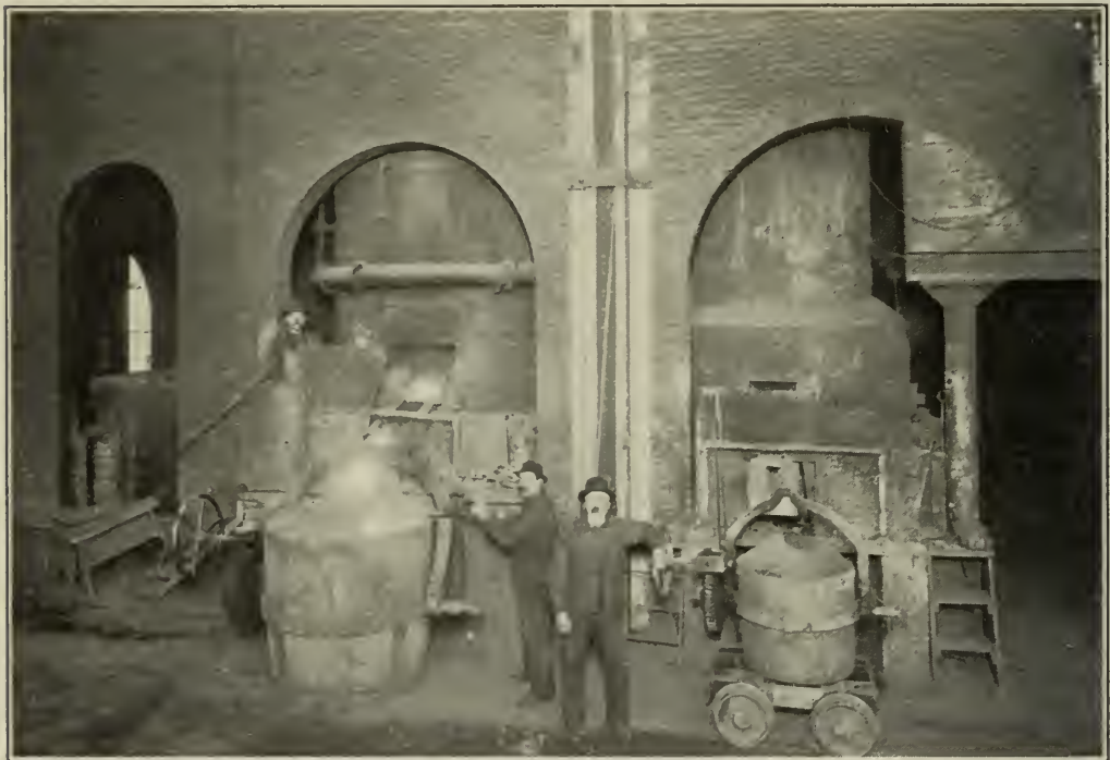
84-INCH COLLIAR CUPOLAS IN RELIANCE FOUNDRY, ALLIS-CHALMERS CO.
